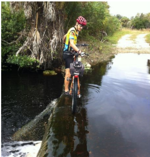
Low water crossing over Deer Prairie Creek at the weir.
