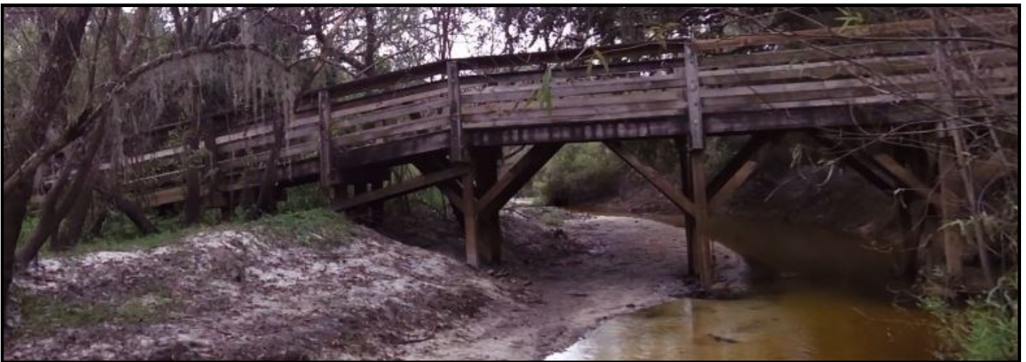
Existing bridge over Myakkahatchee Creek in MCEP.
